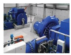
Type of project: Greenfield Scope of service: Complete Solution based on horizontal Francis Turbine.
